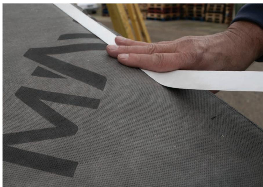
3. Install 50mm PERMAVENT BUTYL TAPE down the rafters to seal any nail penetrations and install counter battens on top of the rafters.
