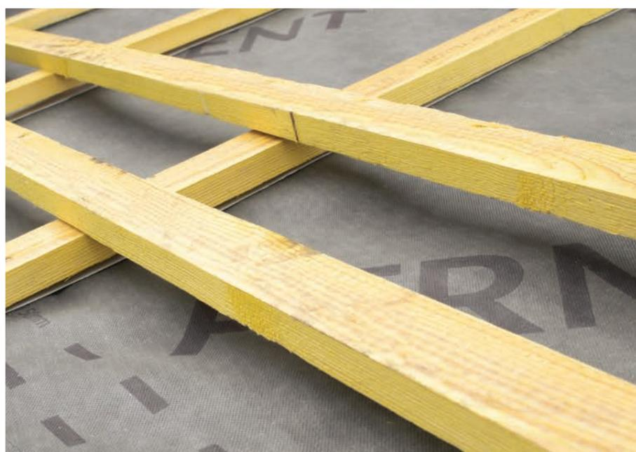
4. Install battens on top of counter battens and lay next layer of PERMAVENT DRY+ with a 225mm head lap so the two adhesive strips meet.
