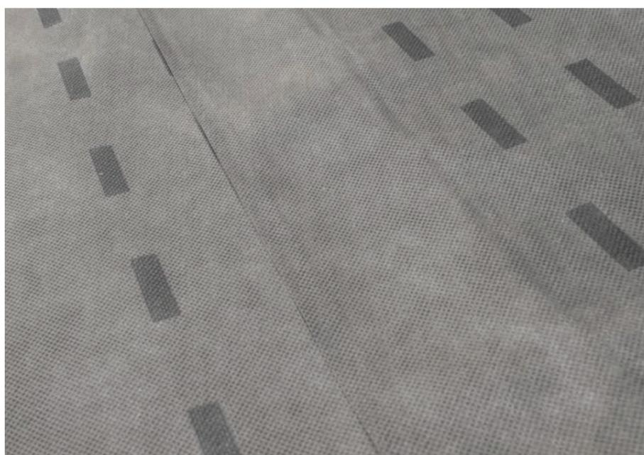
5. Peel back adhesive tape on the two strips sticking the two layers of PERMAVENT DRY+ together.
