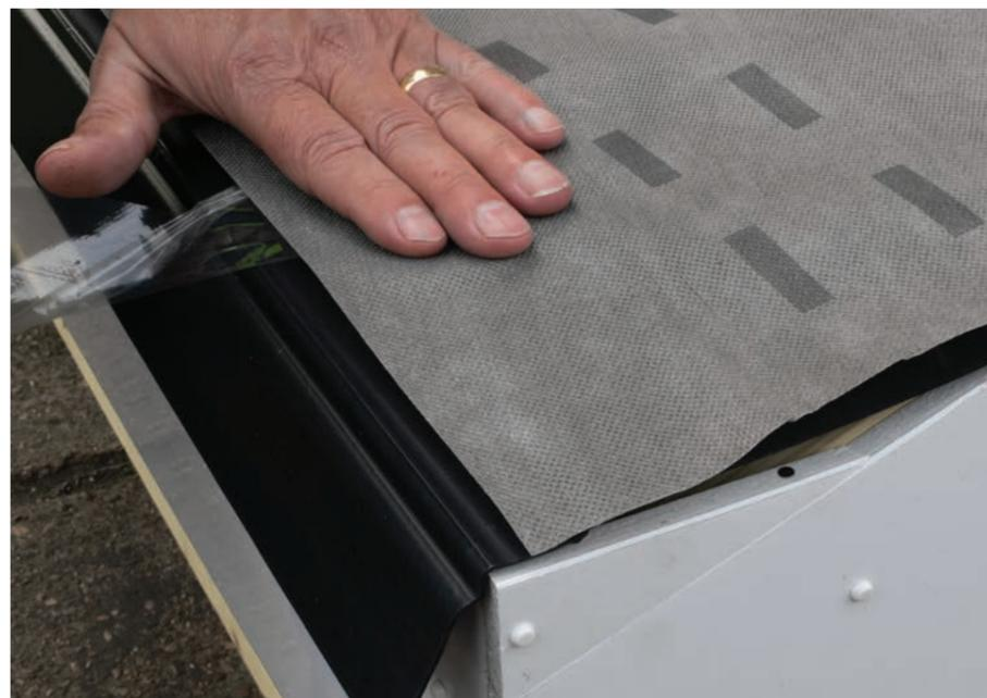
2. Pull off PERMAVENT DRY+ adhesive tape cover and adhere to the membrane support tray.
