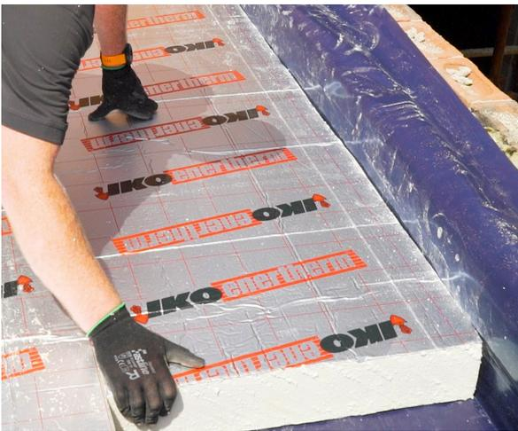
2. The boards should be secured using washers supplied with kit along with additional countersunk screws to suit depth of insulation required.
