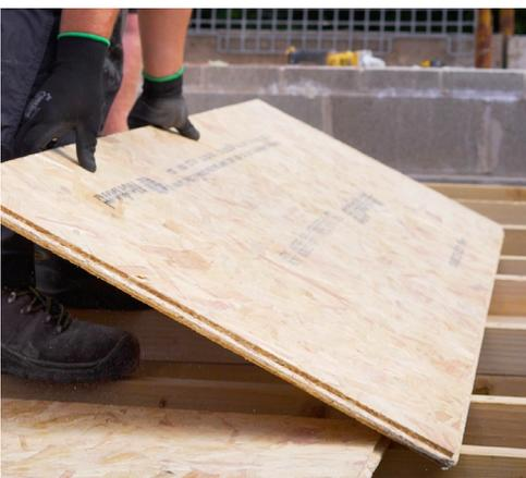
3. Start laying the new row of boards ensuring you stagger the boards adding more strength to the deck area. It is important that any off cuts should span at least two joists.
