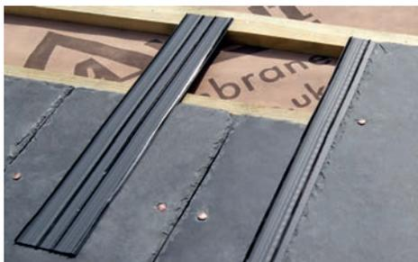
4. When Easy Slate is in position, nail the slate down as normal. This secures Easy Slate in place.
