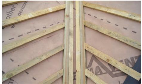
There should be no more than a 20mm gap between a wall and the end rafter. If any larger the membrane can fall down the gap. To prevent this, fix the membrane to the abutment with Permatac double sided tape.
