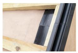
Permavent Easy Verge & Easy VergeTrim products should be installed in conjunction with continuous substrates, such as uniform rafters or softwood sarking. If there is a change-of-elevation or traditional eave-sprocket within your design, please contact our technical team for further guidance.
