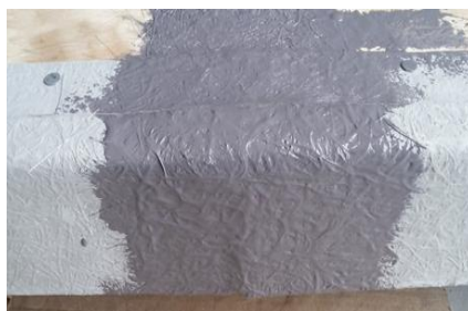
Double reinforced trim joint
