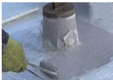
Local reinforcement to stanchion
